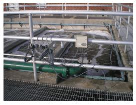
An IQ SENSOR NET module mounted tank side along with sensors for continuous process monitoring and control.
